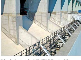
Coke wharf protected with KALCERAM-K on the sliding surface, with KALSICA-N in the zone of high wear and with KALMETALL-C in the area of impact stress
