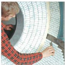
KALOCER mosaics of 1.5 to 12 mm allow flexible use; they are fixed by KALFIX epoxy setting compound
