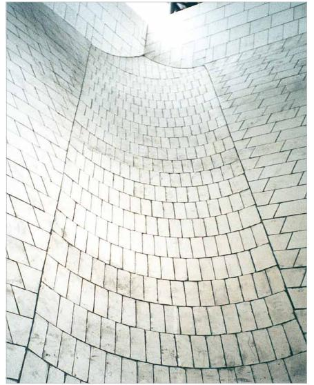
Skip collection chute with KALOCER lining installed at a European blast furnace plant; the shaped elements are up to 50 mm thick and some have been cut three-dimensionally
