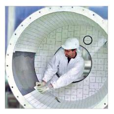
Lining a cyclone inlet with KALOCER; the arch shape enables fixing radial shaped elements in KALFIX setting compound whereas the headwall requires mechanical fixing by means of weld sleeves and ceramic caps
