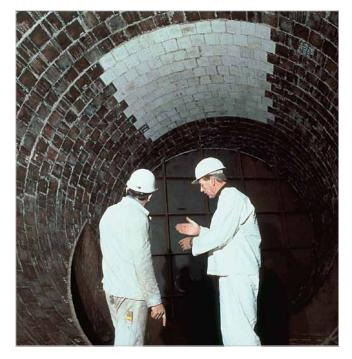
Abrasive sinter particles impinge on the KALCOR lining at 250  $^{\circ}$ C / 482  $^{\circ}$ F and at high velocity – combined with ABRESIST results in an economical solution
