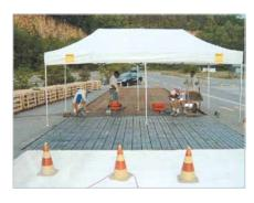
Fused cast basalt has performed well on automobile test tracks all over the world. Here, skid tiles are laid in Switzerland.
