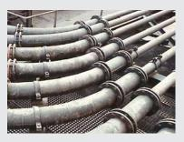
To reduce the severe abrasion of the bends in pneumatic systems, abrasion resistant piping components with internal linings – such as ABRESIST – should be used.
