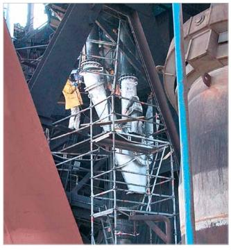
Pressure equalizing pipe set up near a blast furnace; the base metal has a thickness of 30 mm, the thickness of KALMETALL-W 100 hard overlay welding measures 6 mm; 450 mm diameter
