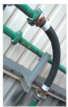
KALFLEX used as flexible pipe bend
