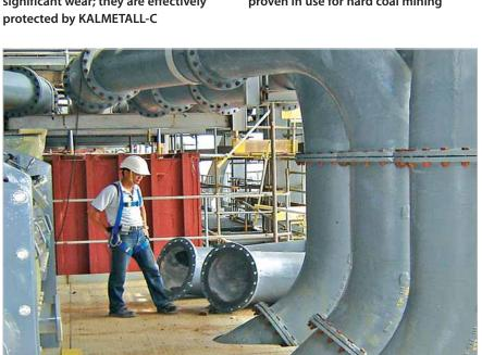
Typical applications of KALMETALL-C hard casting are pipe systems; here a pulverized coal pipe of a power station in South East Asia
