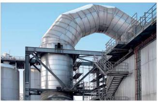
Sinter dust transport pipe in a German cement plant
