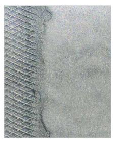
Reinforcement and wire mesh, smooth surface
