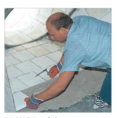
KALCOR lining of a hopper in the sinter dust collector of a steel mill
